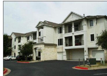
Bridge at Asher
