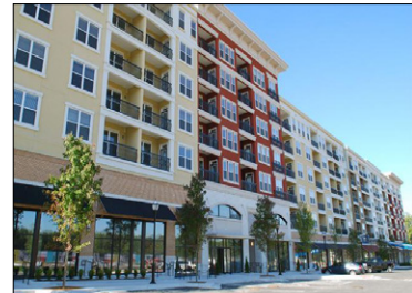
GoodWynn at Town: Brookhaven
