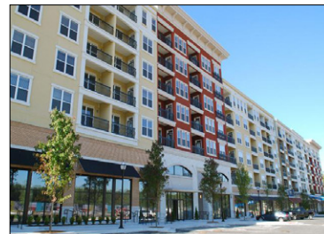
GoodWynn at Town: Brookhaven
