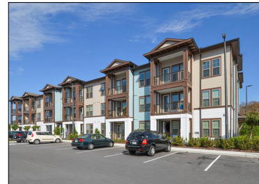
Lantower Grande Flats
