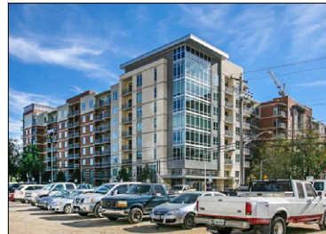
Camden Rainey Street
