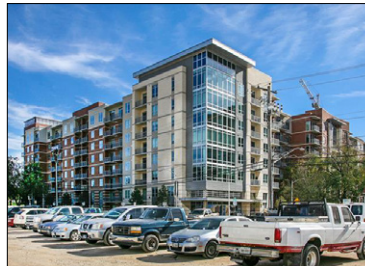
Camden Rainey Street
