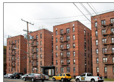
29-32 Beach Channel Drive
