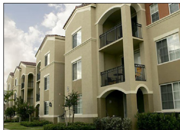
Milano at Miramar
