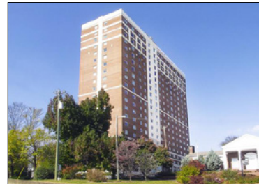
The Tower at Morgan Hill
