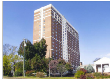
The Tower at Morgan Hill
