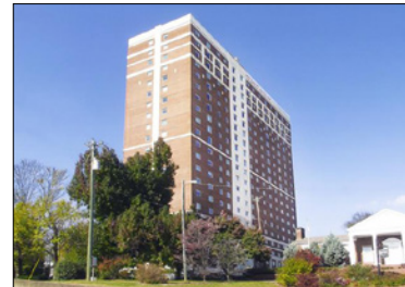
The Tower at Morgan Hill
