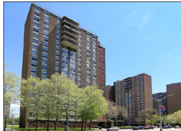
Spring Creek Towers
