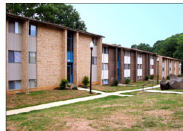
Gwynn Oaks Landing
