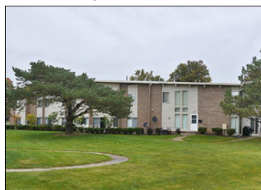
The Crossings at Canton
