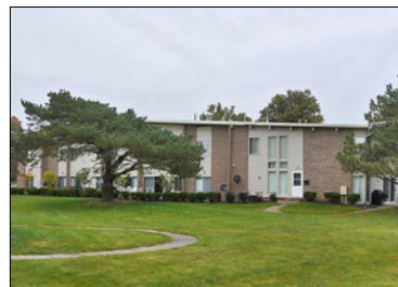
The Crossings at Canton
