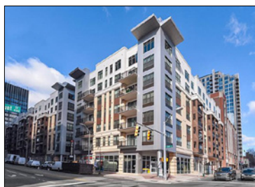
The Edison Lofts
