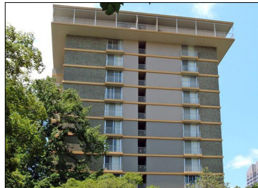
Capitol Towers and Villas
