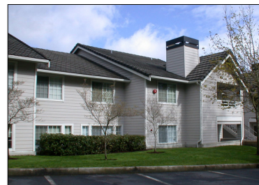
Overlook at The Lakemont
