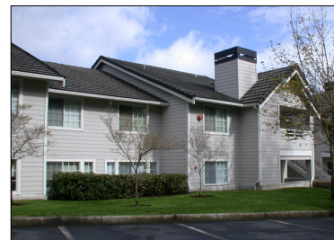
Overlook at The Lakemont
