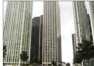
North Harbor Tower
